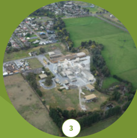
AERIAL VIEW OF THE TRARALGON LIME PLANT IN VICTORIA, AUSTRALIA
