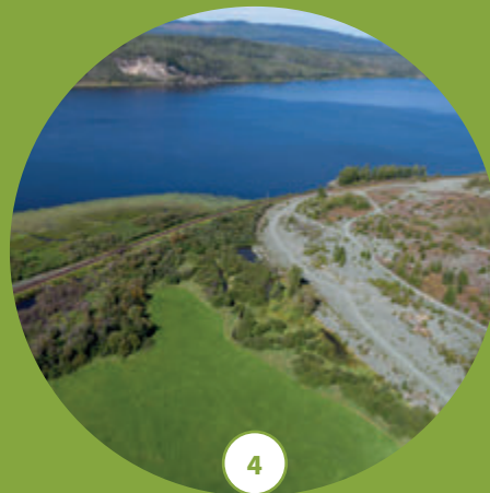
AERIAL VIEW OF THE GISCOME PROJECT SITE IN BRITISH COLUMBIA, CANADA
