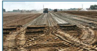
from this reaction further dries wet soils. The reaction with water occurs even if the soils do not contain significant clay fractions. When clays are present, lime's chemical reactions with clays increase the moisture-holding capacity of the soil, which reduces free liquids and causes further drying.
