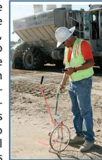
Lime addition of three to six percent by mass of the dry soil is the customary range for lime stabilization in road foundations. Precise amounts should be determined through mix design and testing protocols.
