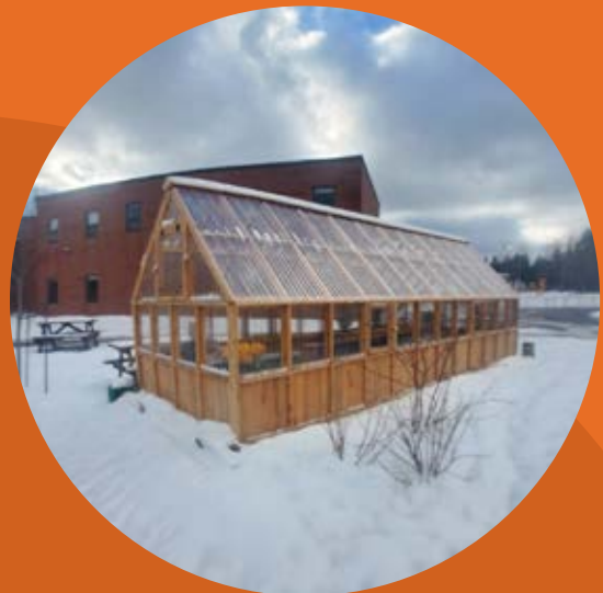
Greenhouse at Petiscodiac High School built on top of stone donated by our Havelock, New Brunswick Plant
