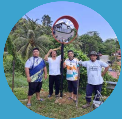
Convex mirrors installed to provide better visibility at problematic intersections
