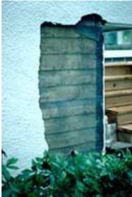
The stucco will be applied to the wire lath laid over the area to be patched. Photo: NPS files.
