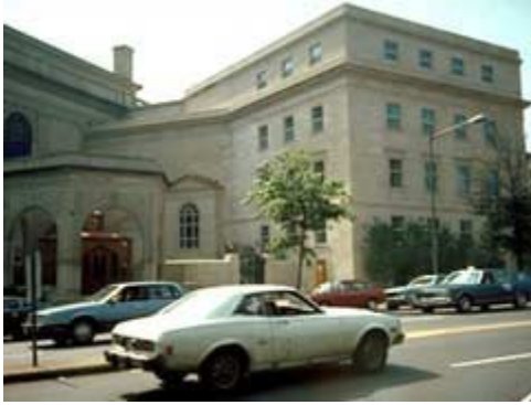
The new addition on the right is stucco scored to imitate the limestone of the historic building on the left. Photo: NPS files.
