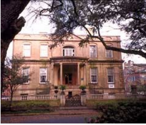
The stucco on the early-19th century Richardson-Owens-Thomas House in Savannah, Georgia, is a type of natural cement. Photo: NPS files.
