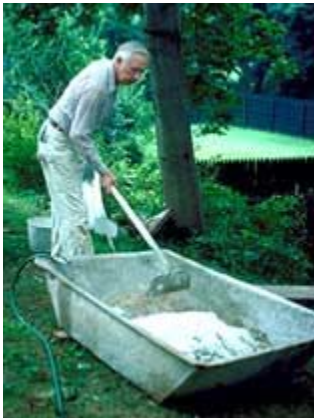
The dry materials must be mixed thoroughly before adding water to make the stucco. Photo: NPS files.
