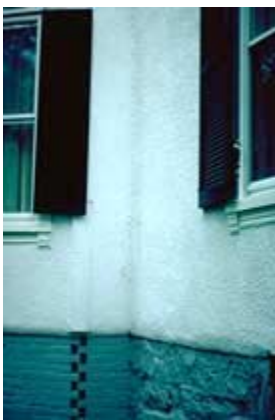
This stucco house has a rough cast finish. Photo: NPS files.
